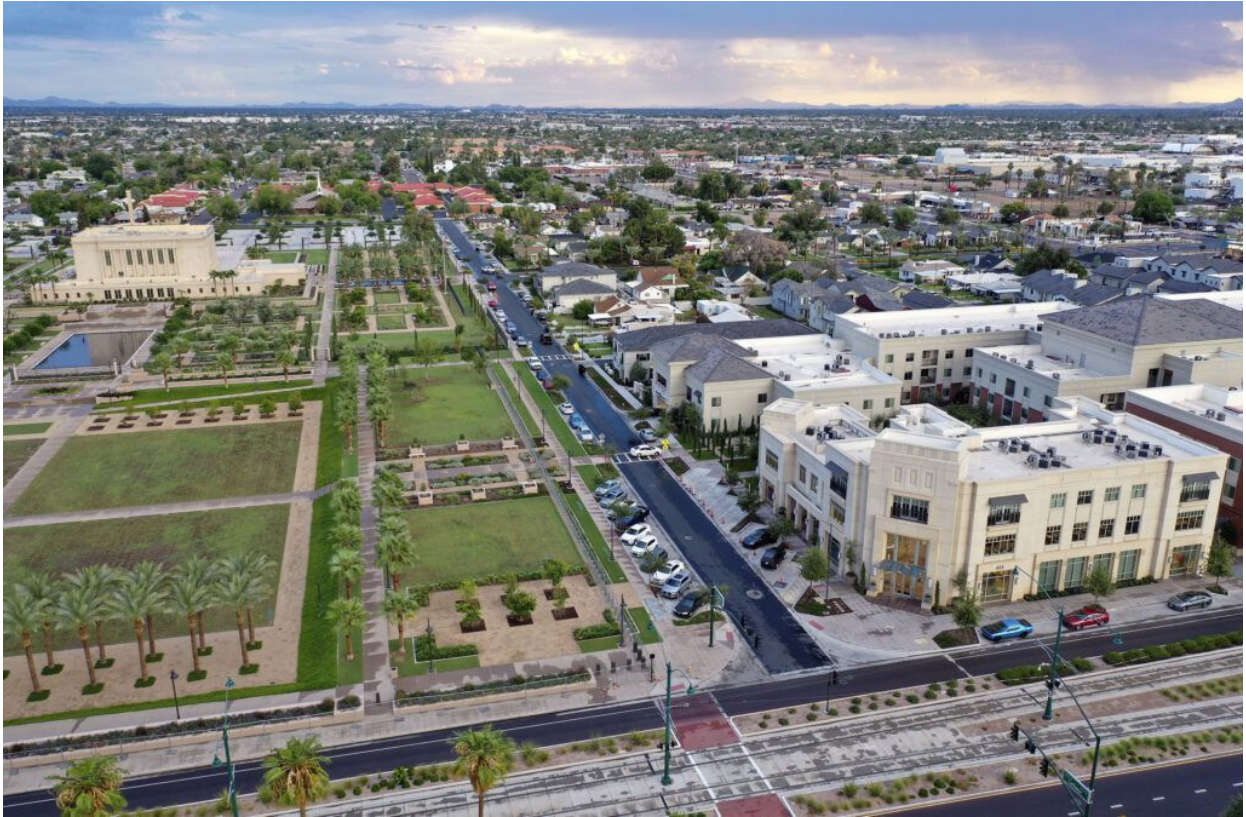
View of redevelopment next to light rail tracks on Main Street – Photo Credit: LDS Church (Church of Jesus Christ)
