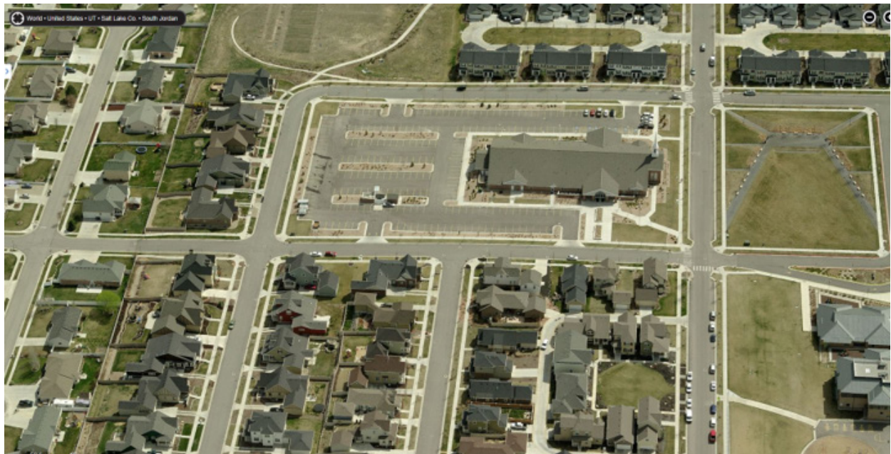
2000 Church of Jesus Christ of Latter-day Saint Chapel located in Daybreak, Utah on 4.3 acres with 247 onsite parking spaces despite community's walkability. Image: Bing Maps
