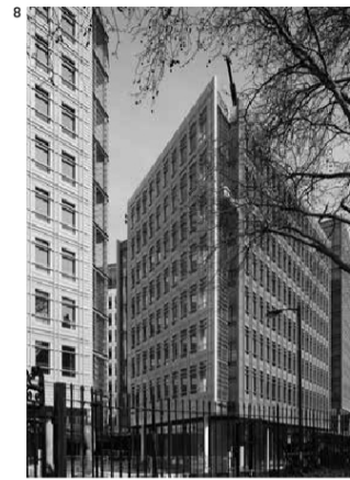
8. The gaudy glazed ceramic facades of Renzo Piano's Central St Giles mixed-use complex have created a clumsy conflict between new and old in London
