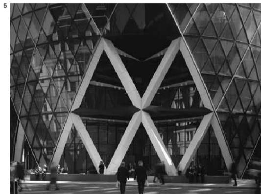
4. Although it is a masterpiece of computer modelling and highly specialised environmental design, Foster + Partner's 50 St Mary Axe does little to engage with its surrounding context 5. The innovative diagrid efficiently uses 20 per cent less steel than a conventional rectilinear block
