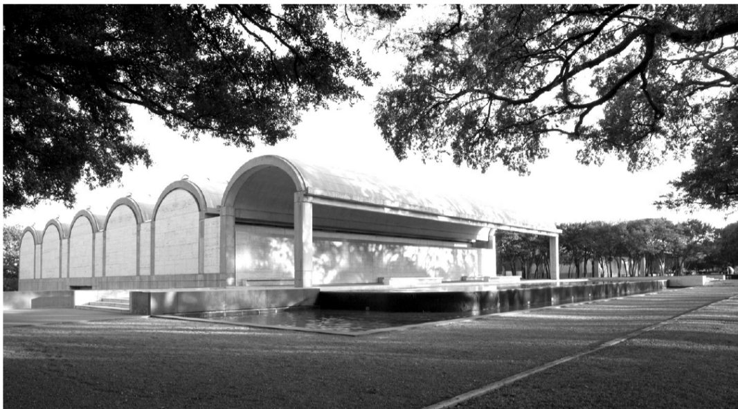
Kimbell Art Museum by Louis Kahn 32. View from park with vaulted porch leading to entrance court and grove 33. Entrance lobby 34. Typical view of gallery 35. Plan 36. Section
