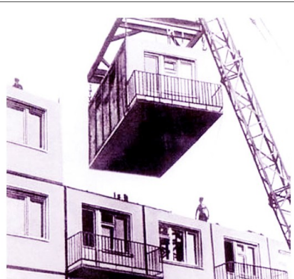
Figure 8 - modular design and assembly of Khrushchevka-style apartments (Markin, 2019)
