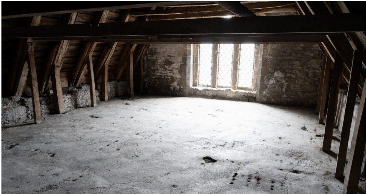
Fig. 13 - Tracing floor at Wells Cathedral Cloister: A tracing floor is a room set aside in the jobsite where the floor is covered in thin plaster. The master mason would draw building elements through scratching the plaster, laying out precise measures using the compass. This was used as a template by stone cutters
