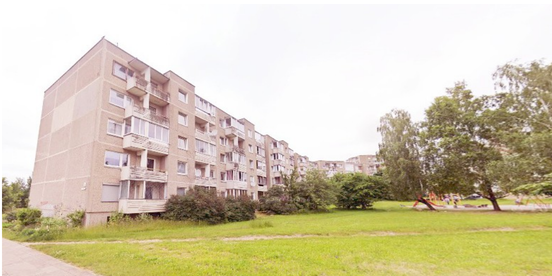
[Fig. 2: Khrushchevka apartment building in Šeškinė, Vilnius, Lithuania, showcasing grid-like concrete facade demonstrating prefabricated concrete panels. (Google, 2025)]
